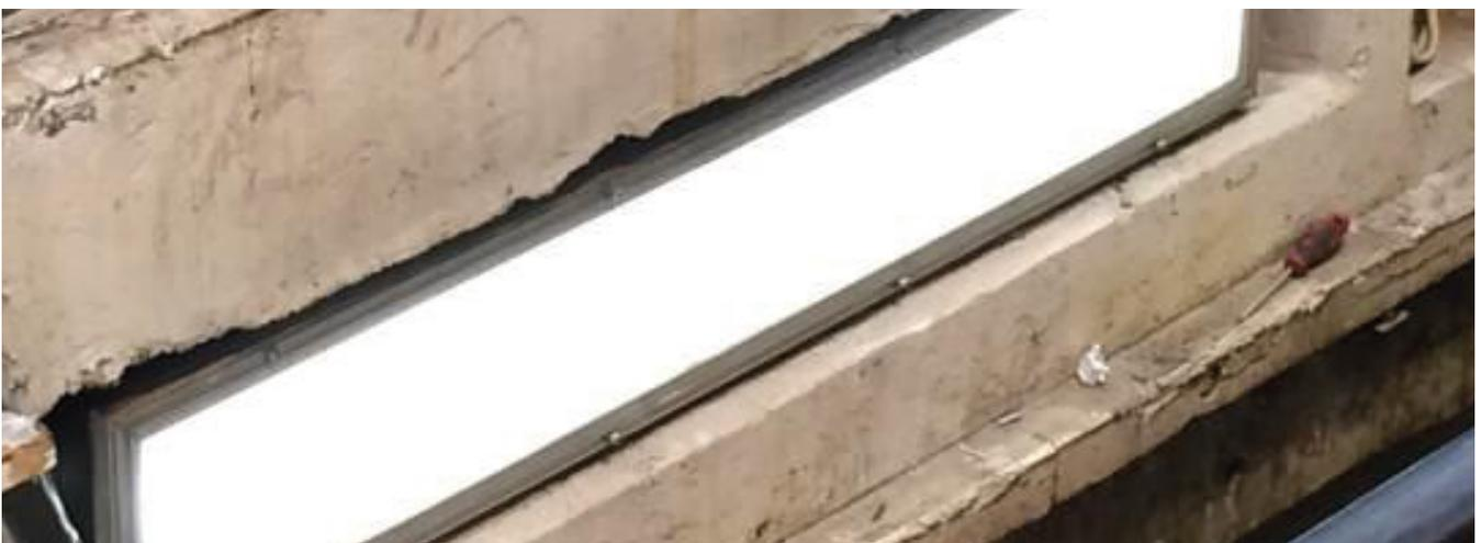
6. Replace the original diffuser above the new LED light source
