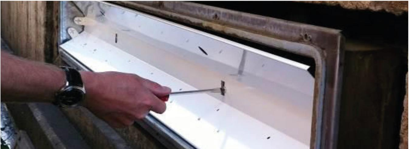
2. Remove the diffuser and the existing reflector plate and ballast
