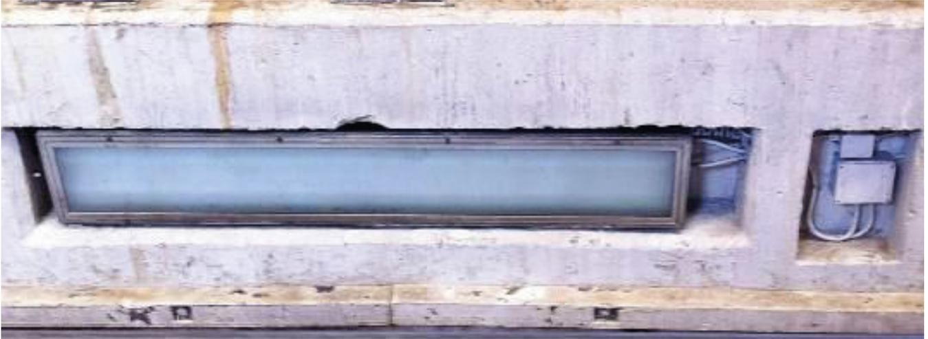
1. The existing fitting in the pit wall equipped with twin T8 fluorescent lamps
