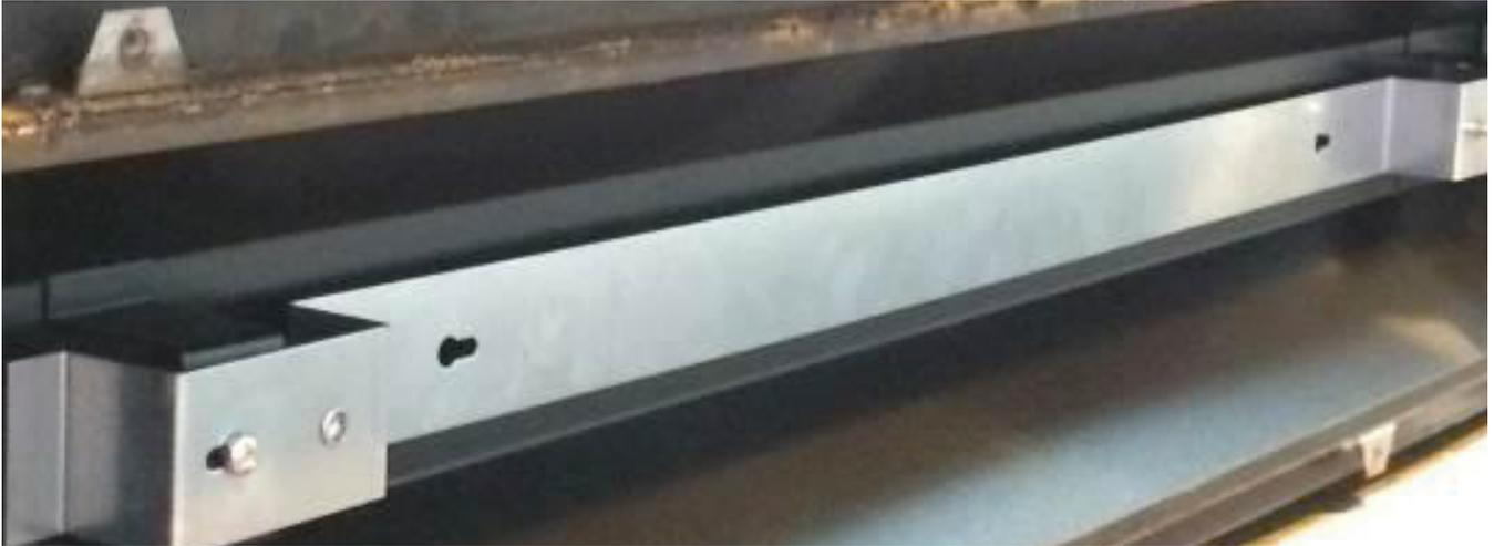
4. Attach the bespoke bracket to the existing carcass (just 2 fixings)
