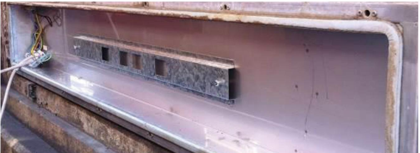
3. The existing bracket (one of two different types found on this installation)
