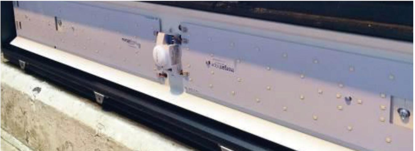
5. Attach the Morgan Hope LED gear-tray to the bespoke bracket (just 2 fixings)
